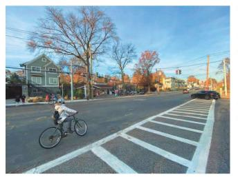
Cyclists traveling to this intersection along Boston Post Road are forced to cross the commercial driveway at the fuel station during permissive northbound Boston Post Road signal phase. Ideas include making it a protected-only signal phase, prohibiting left turns into that driveway, and closing the driveway (there are two other driveways to enter/exit this commercial business if the third was to be closed).
